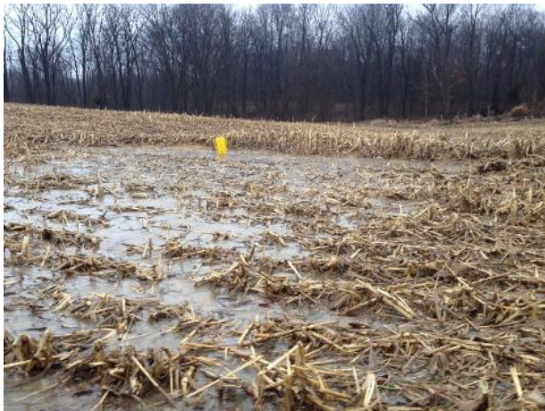
Surface riser in depression, with potential for residues and sediment to enter tile drain system through surface runoff.
