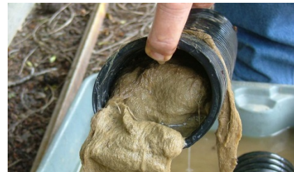
Roots and sediment clogging tile drain.
